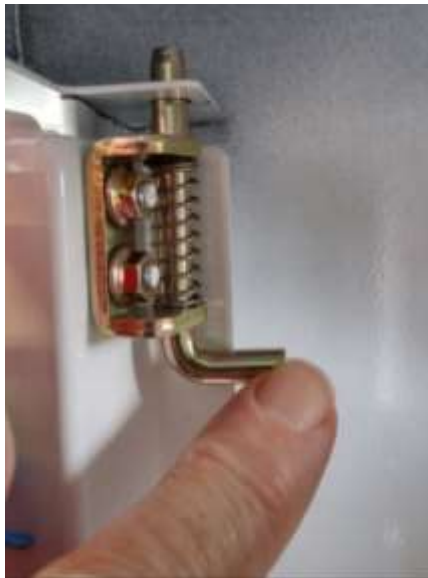
Pull down the top-hinge pin
